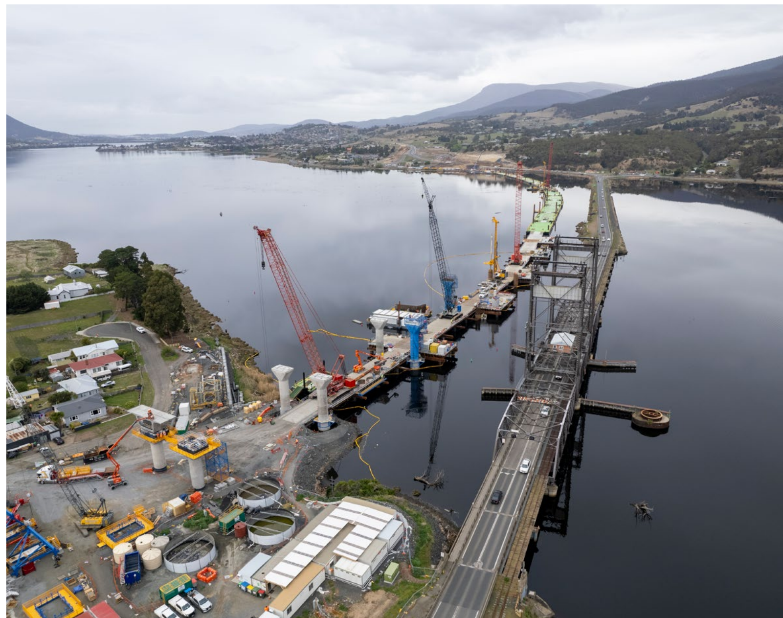
Temporary bridge access over the deeper water channel.
