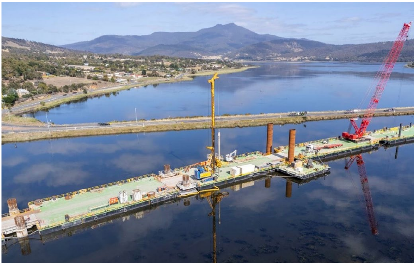
Grounded barges for access over the mud-flats (causeway in the background).
