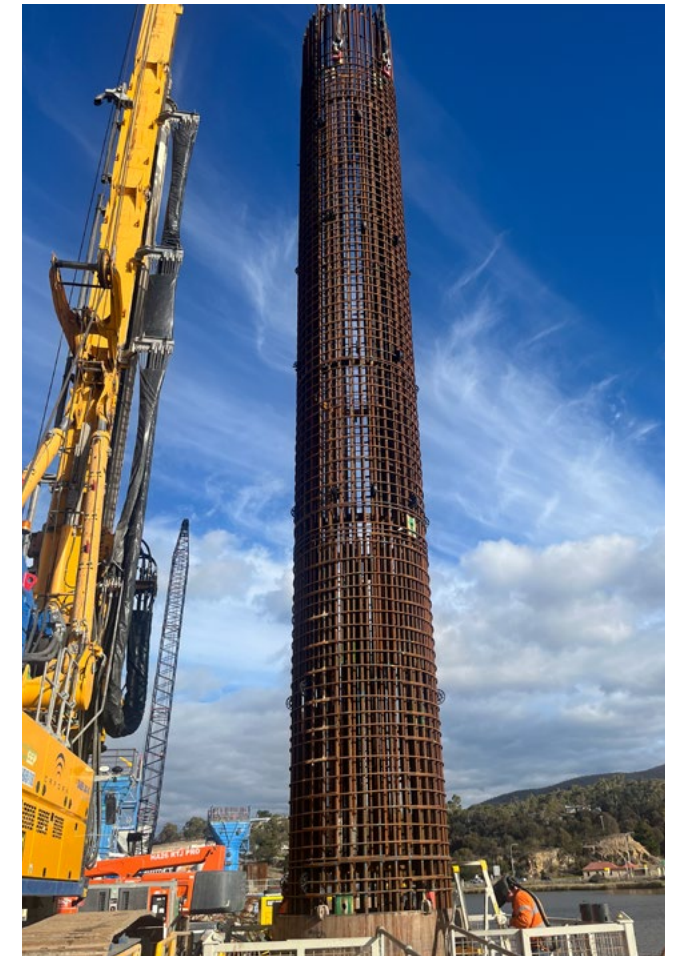
Reinforcement cage installation.
