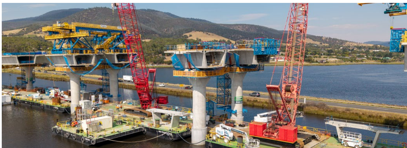
The pier head segments were erected by crane, while the field segments were lifted into position by the Special Segment Lifting Devices.
