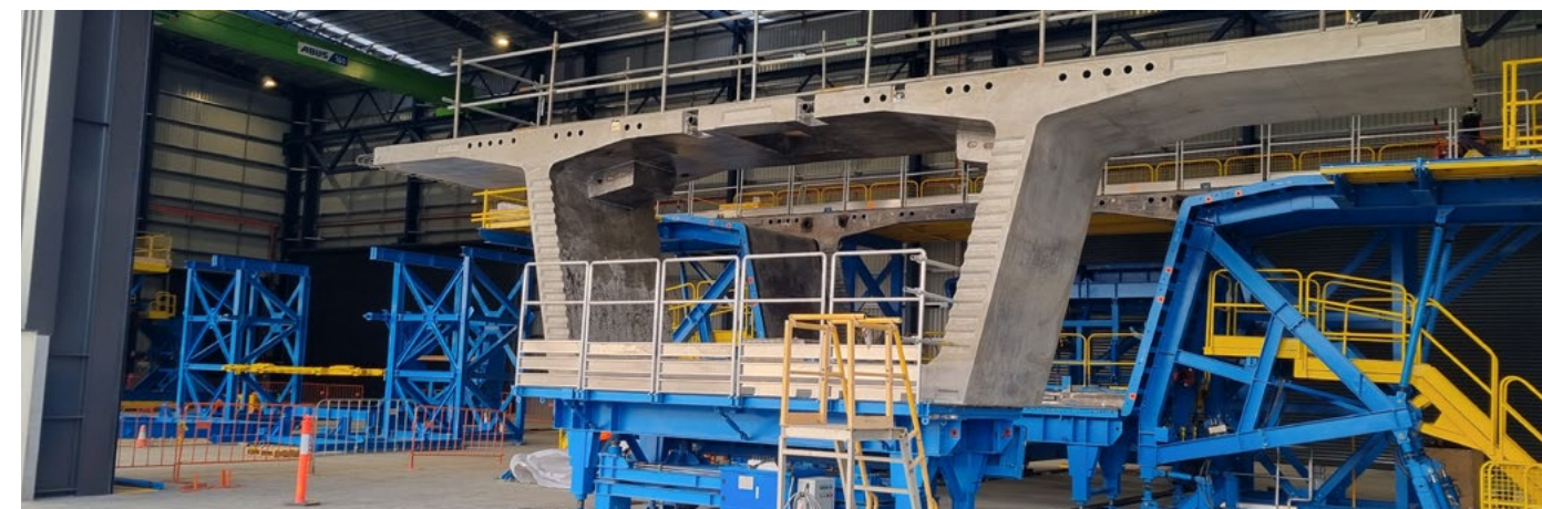
A segment has been cast from the mould at the bespoke pre-cast facility.
